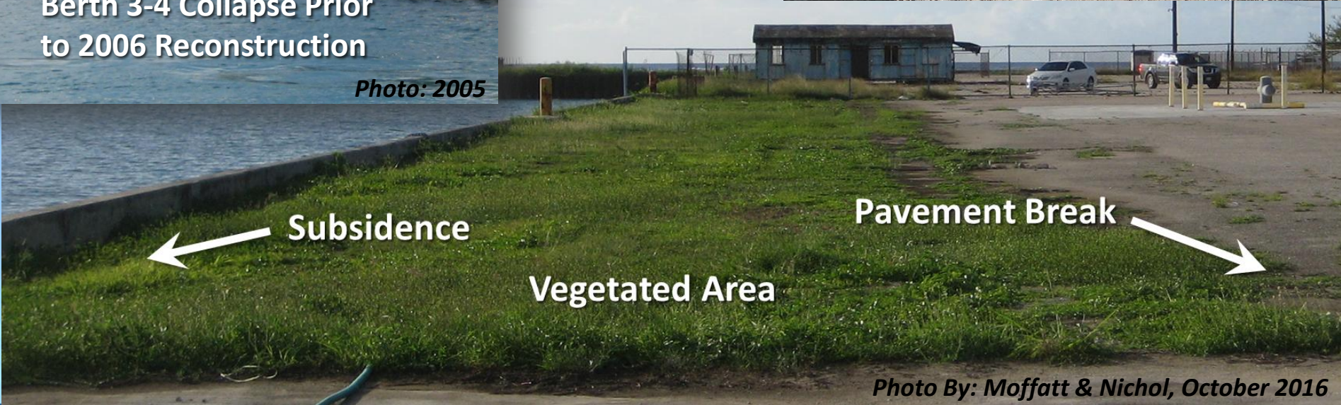
4 to 8 inches of pavement subsidence
